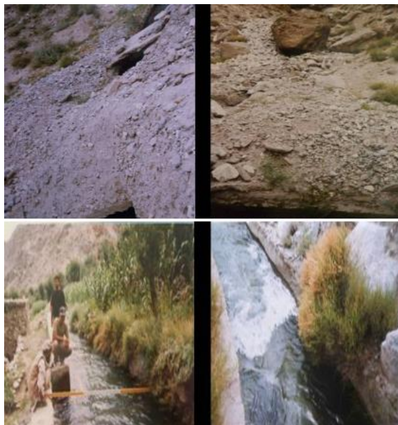
Fig. 3 Reduction in cross-sectional area of power canal.
