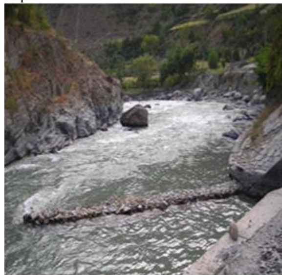
Fig. 1 Existing view of temporary stone weir
