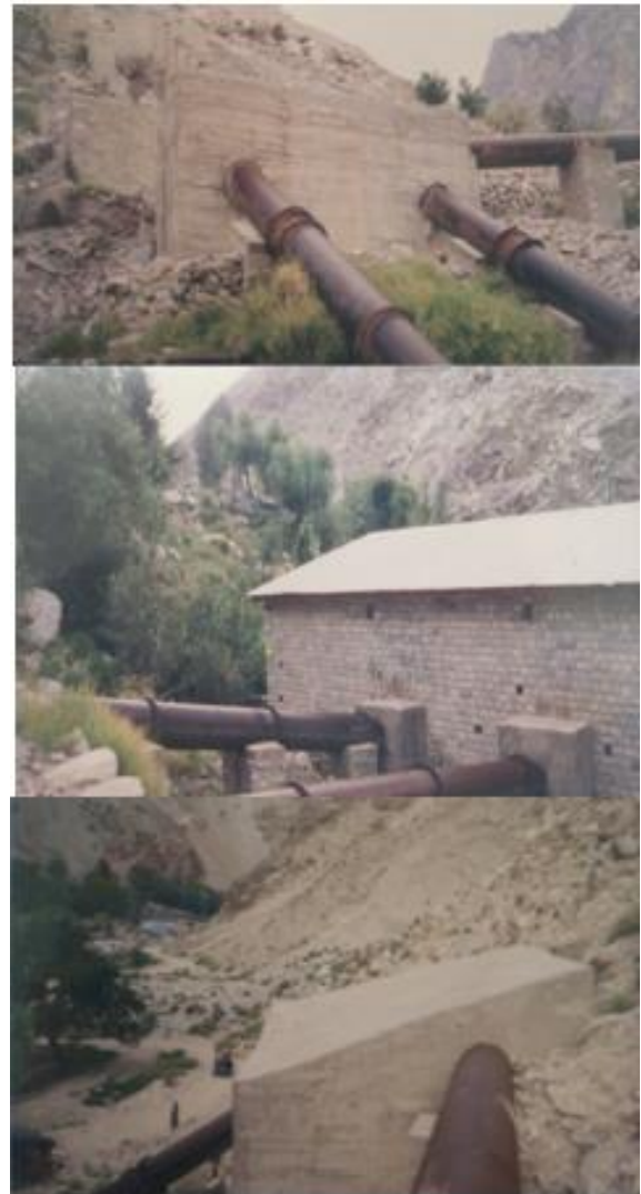
Fig. 5 Splitting of one penstock into two.
