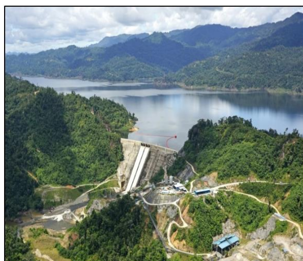
Fig. 2 Murum Dam in Sarawak state of Malaysia
